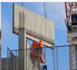
Façade installation commences on the external walls – the first of 1200 concrete panels.
